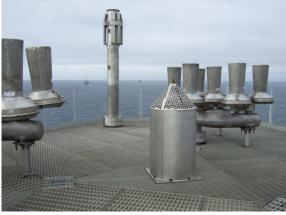
The UK North Sea Forties field offshore flare platforms required replacing in 2007, as they had been in situ since installation in 1976. Locker Heatshielding were contracted by Amec to provide replacement Heatshield panels for the Forties Alpha flare platform to protect the Flare deck structure from elevated temperatures.
