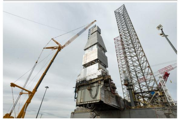
**Transocean Galaxy 1** was selected for a drilling campaign on the Elgin field within the North Sea as a direct replacement for the previously operating Rowan Viking Drilling Rig. Due to the close proximity of the drilling rig to the flare boom of the Elgin platform there was a requirement to fully enclose the drilling derrick of the rig, which consisted of placing Heatshields on all four sides, as well as covering the crown block roof.
