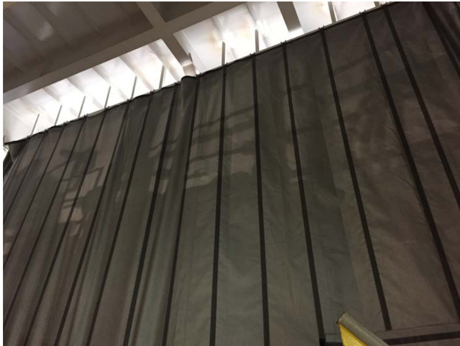
Cantilever panels attached to upper beam using ratchet clamps (view from inside)
