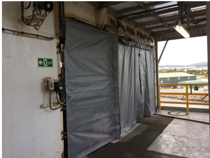
Cantilever panels attached to upper beam using ratchet clamps (view from inside)
